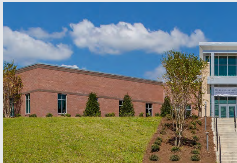
Aiken Technical College Center for Energy and Advanced Manufacturing Graniteville, SC
