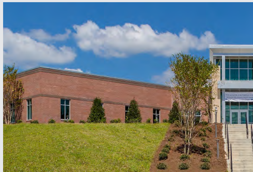
Aiken Technical College Center for Energy and Advanced Manufacturing Graniteville, SC
